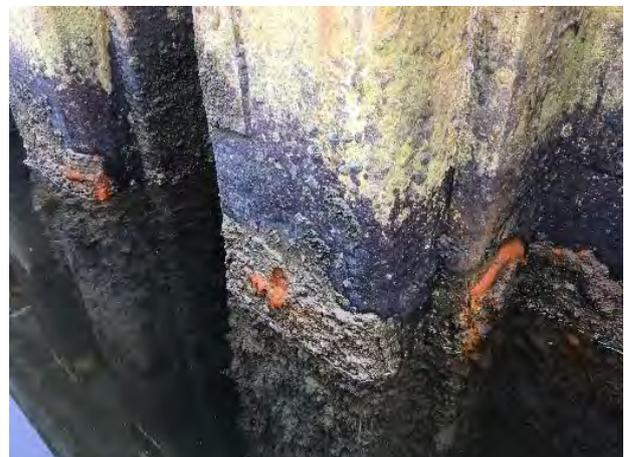
Orange growth/tubercles, typically associated with accelerated low water corrosion is one of the MIC topics studied at Swinburne.
